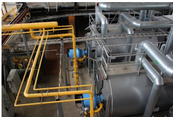
Figure 11 Old fossil fuel fired boiler
