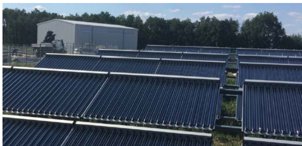
Figure 8 Installed tube collectors
