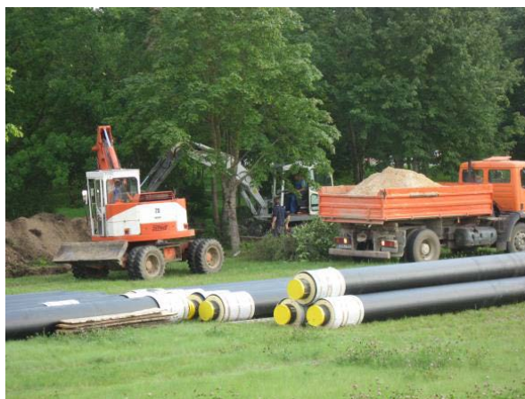
Figure 17 New cased underground pipelines
