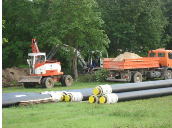
Figure 17 New cased underground pipelines
