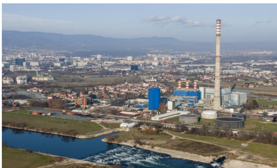
Figure 2 Thermal power plant of Zagreb with the new, integrated thermal storage (blue),
