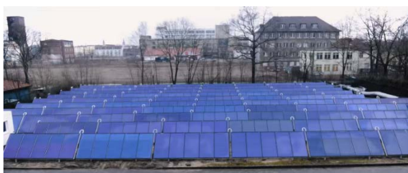
Figure 22 After the retrofitting measure (source: Vattenfall Deutschland )
