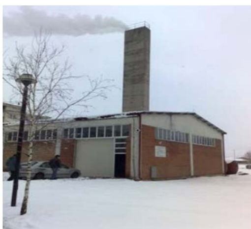
Figure 18 Before the upgrading process
