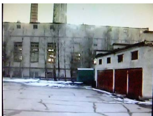
Figure 14 Before the upgrading process
