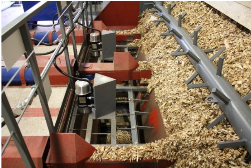
Figure 13 Feed-in system of a woodchip boiler
