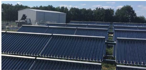
Figure 8 Installed tube collectors
