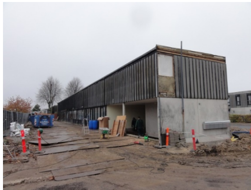
Figure 24 During the upgrading process
