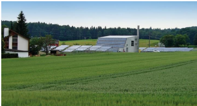
Figure 34: Heating plant with solar thermal collectors in the village Büsingen, Germany (Sources: left: Solites; right: D. Rutz)
