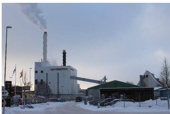
Figure 43: CHP plant of Ena Energie in Enköping using wood chips from waste wood (right) and from short rotation coppice (SRC) (Sources: D. Rutz)
