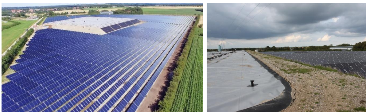
Figure 36: Solar DH collector field in Gram, Denmark, with a seasonal pit thermal energy storage (Sources: left: Gram Fjernvarme, right: D. Rutz)
