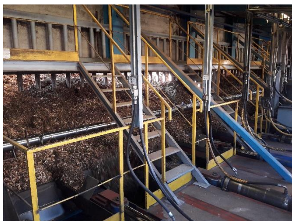
Figure 42: CHP plant in Salcininkai, Lithuania, in which a biomass boiler (5 MW th ) replaced one of the three natural gas CHP units. The remaining two gas CHP units have a capacity of 3.5 MW th and 6 MW th (Sources: D. Rutz)
