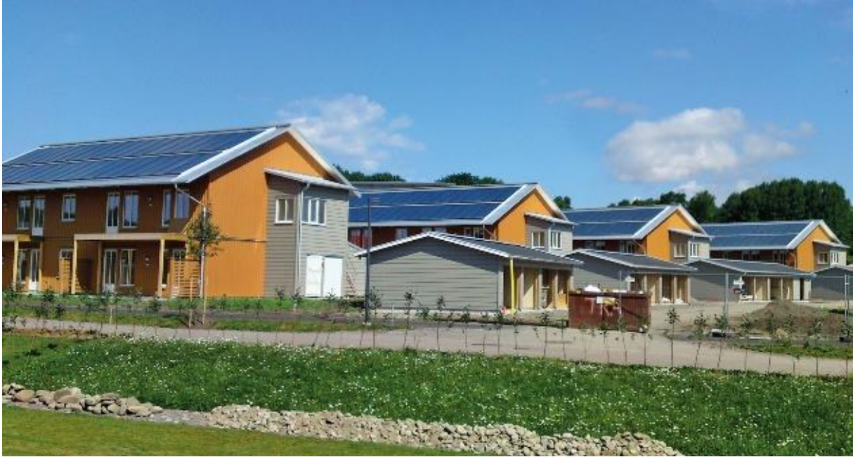
Figure 33: Solar DH in the residential area of Vallda Heberg, Sweden (Source: Jan-Olof Dalenbäck)
