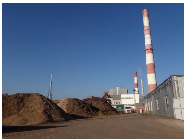
Figure 42: CHP plant in Salcininkai, Lithuania, in which a biomass boiler (5 MW th ) replaced one of the three natural gas CHP units. The remaining two gas CHP units have a capacity of 3.5 MW th and 6 MW th (Sources: D. Rutz)
