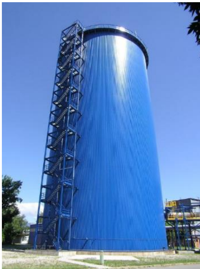
Figure 55: Non-pressurized thermal storage of the DH system in Zagreb (Source: www.pogledaj.to )
