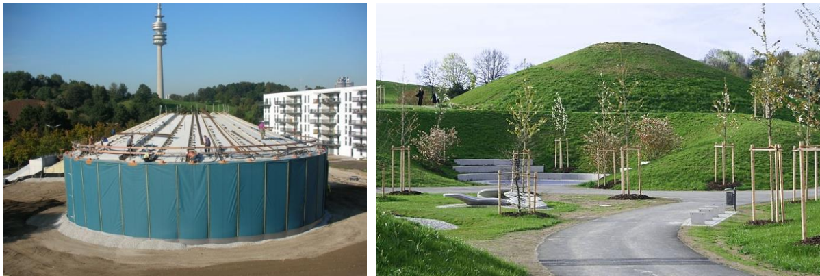
Figure 57: Tank thermal energy storage with 5,700 m 3 of water volume built from prefabricated concrete elements in Munich, Germany (in construction and finalized, Sources: Solites)
